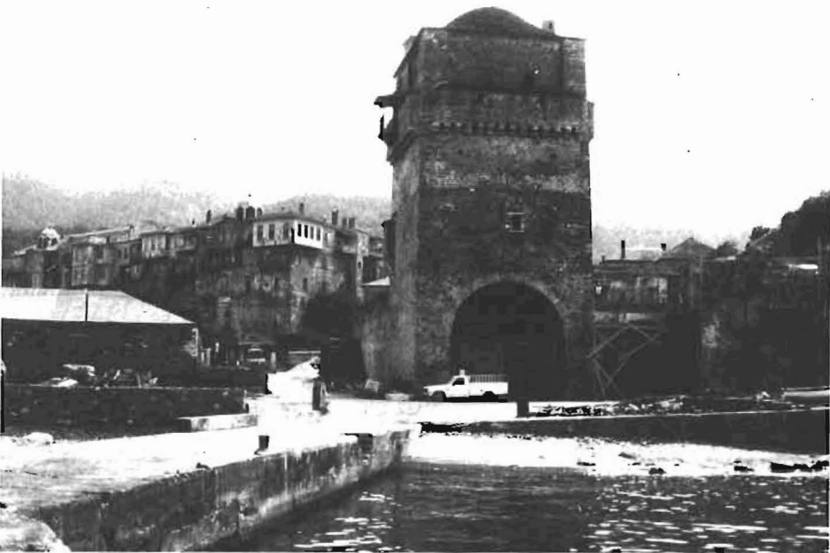
Boathouse. Front View.
